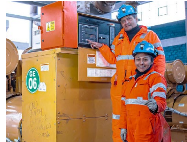
Machine tending at Caylloma Mine
