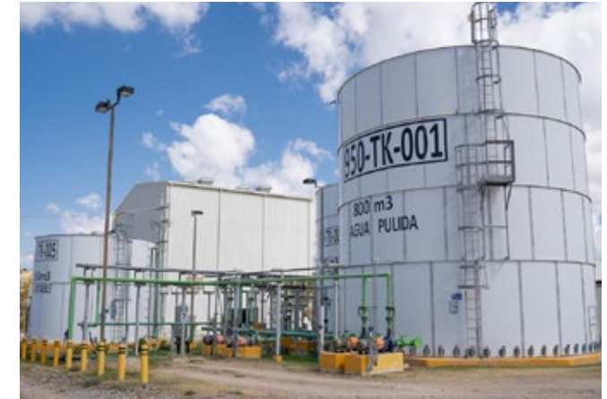
Water tanks at San Jose Mine
