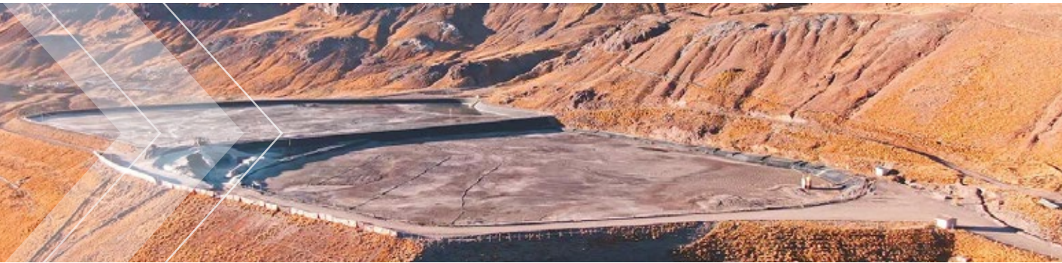
TSF at Caylloma Mine
