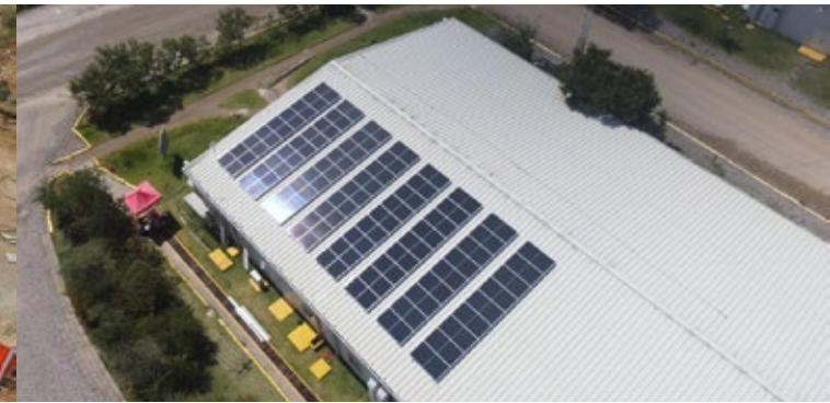
Solar panels on admin building at San Jose Mine
