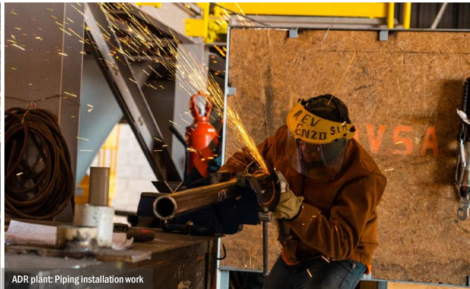
ADR plant: Equipment installation work
