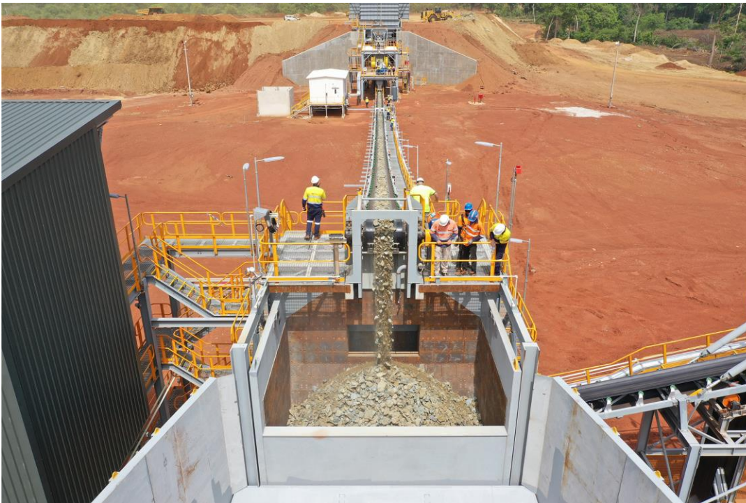
Mineralized material being crushed and conveyed to the stockpile
